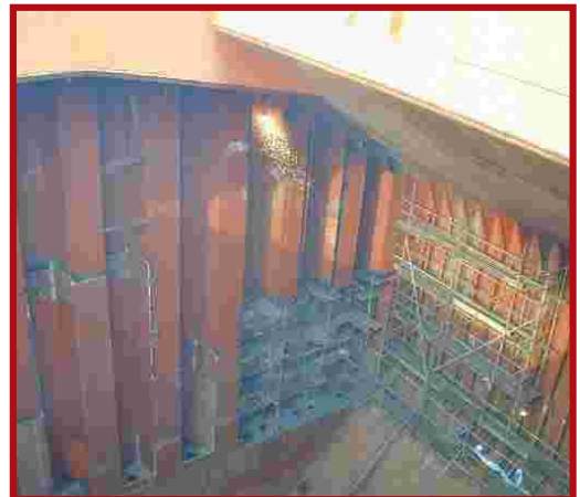
Corrugated bulkhead renewal.
