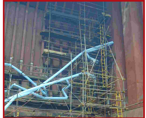
Renewal of side shell frames and brackets.
