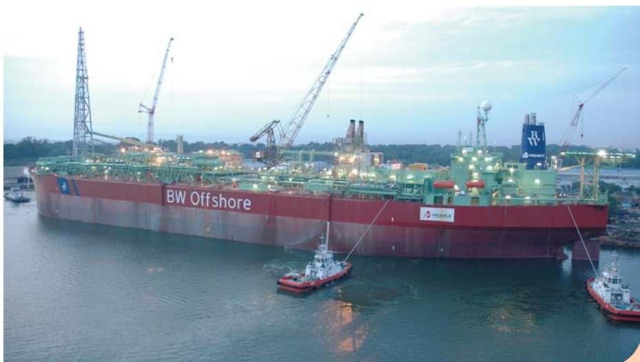
A newly completed YÜUM K'AK'NÁAB sailing off for her maiden deployment in Gulf of Mexico
