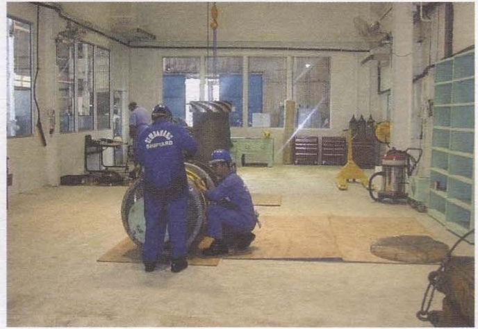
Fully airconditioned cryogenic workshop.
