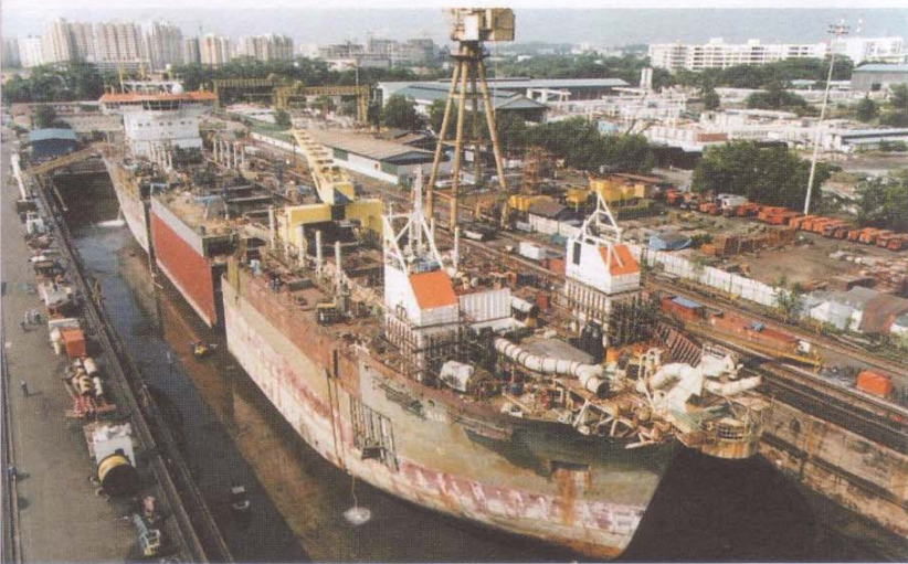
Lengthening work in progress.
