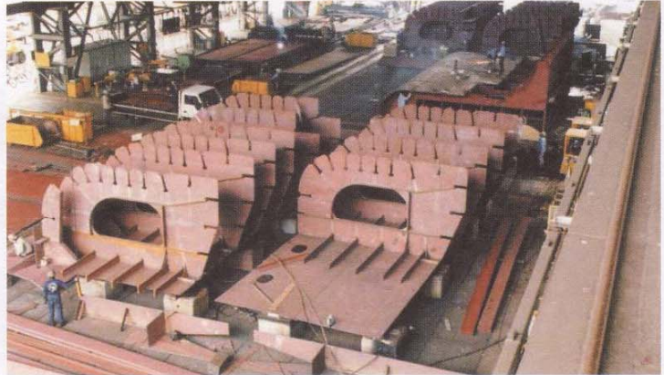
Extensive fabrication work carried out in our steel workshop in Sembawang Shipyard.
