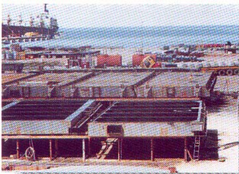
Hatchcover Fabrication (Stage 1) requiring 850T of steel
