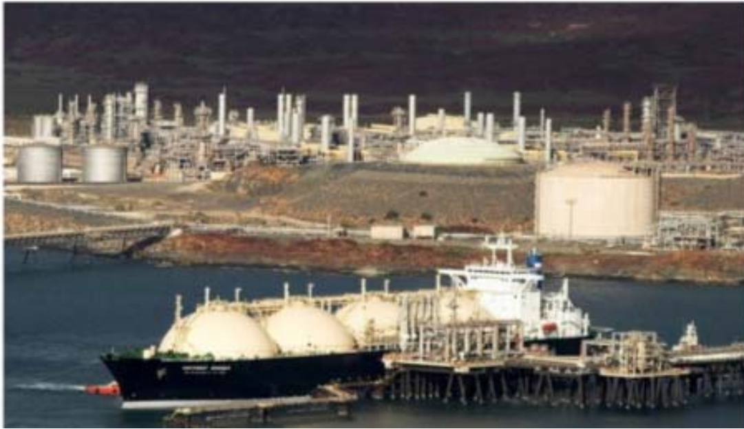
NWSSSC's LNG (in the foreground) and Karratha Gas Plant (in the background).
